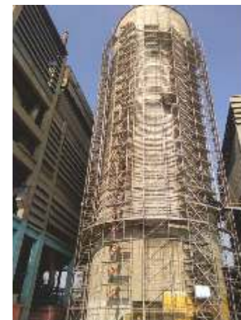
Layher Allround Scaffolding with Aluminium platform stairway up to 48 mtr height at Cement Plant in Panipat, Haryana India (Courtesy: BBN Engineering)
