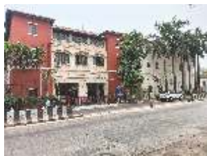
Heritage Facade Restoration
